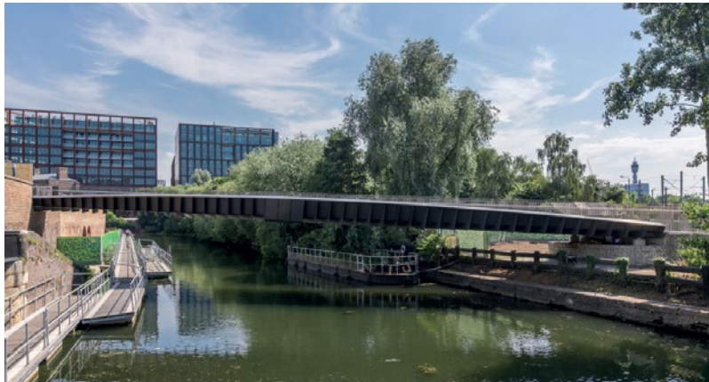
Somers Town Bridge Moxon Architects 38 metres 2017
