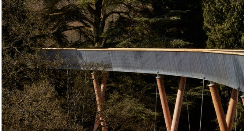
Westonbirt Tree Walk Glenn Howells Architects & Buro Happold Engineering 284 metres 2016 £1.9 million £3500/m2 construction cost
