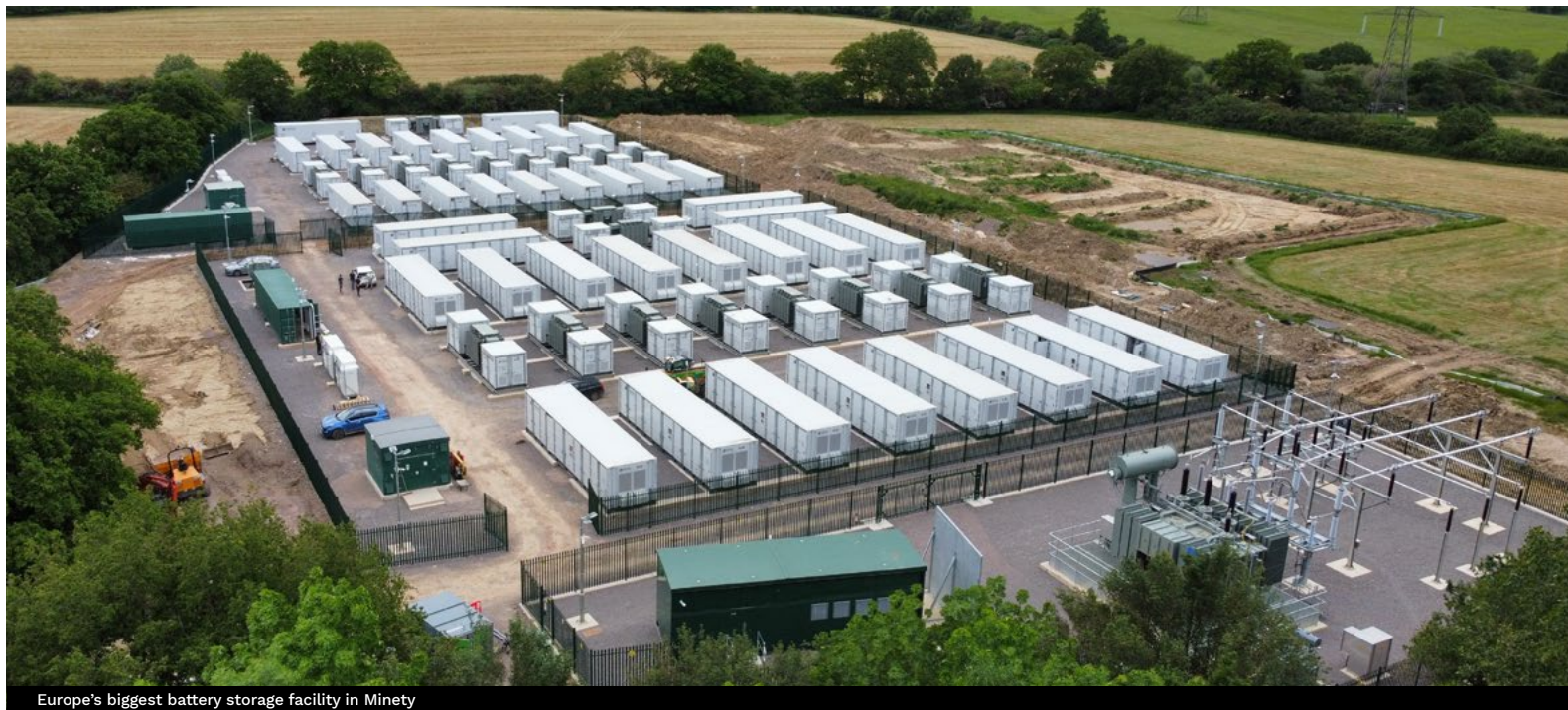
Europe's biggest battery storage facility in Minety
